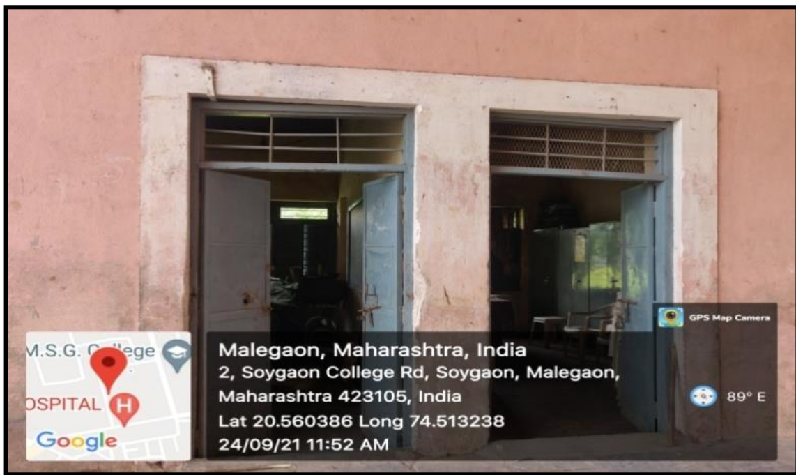
Entry Gate -Gymkhana
